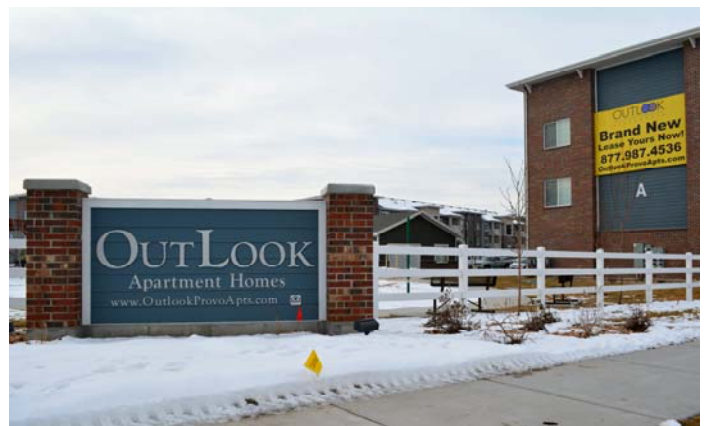
Figure 10 Outlook Apartments at 664 S. 2600 West
