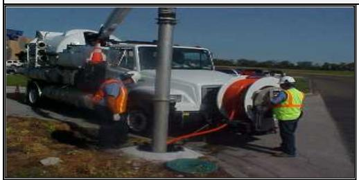
A storm drain is "flushed" with water to suspend and remove deposited materials. Flushing is particularly beneficial for storm drain pipes with grades too flat to be self-cleansing. Flushing helps ensure pipes convey design flow and remove pollutants from the storm drain system.
